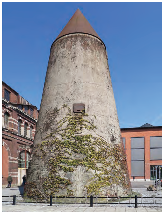
Malmö’s Spitzbunker of cast concrete and an iron-coned roof has protected status reflecting its rarity
